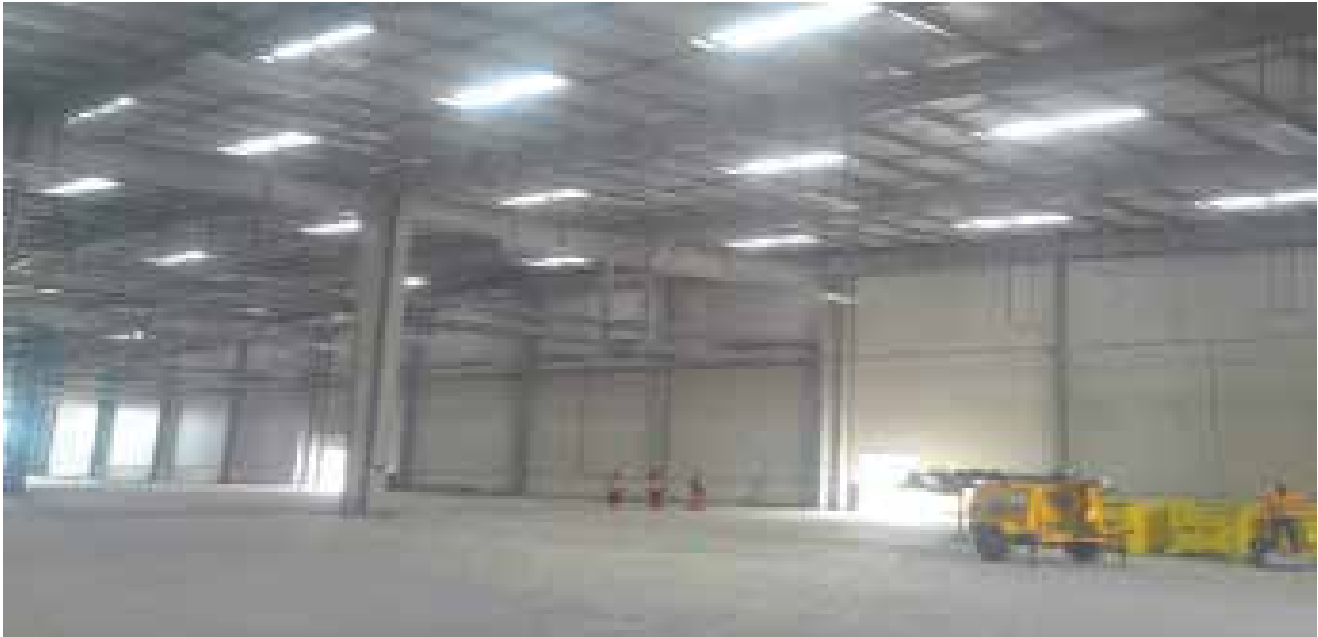
Actual image of work in progress
